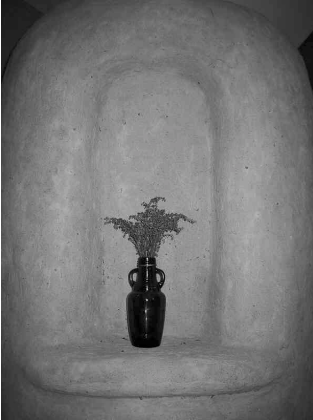
photo: earthen niche in a masonry heater
