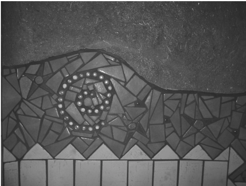
photo: recycled glass & salvage tile scraps on a cob wall
